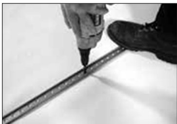
Installation des rails Sarnafasteners
