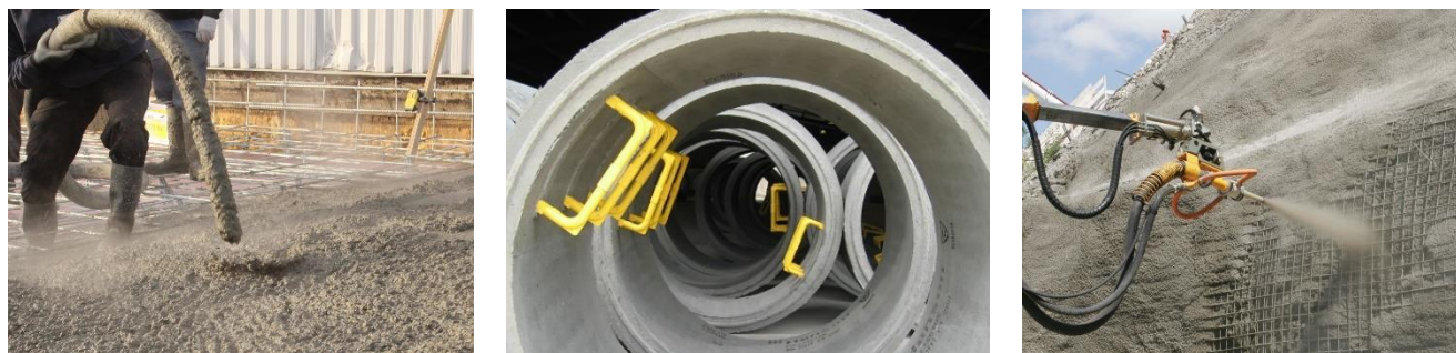
Figure 1: Applications for concrete admixtures (from left to right: air entrainer, dry cast and set accelerator)
