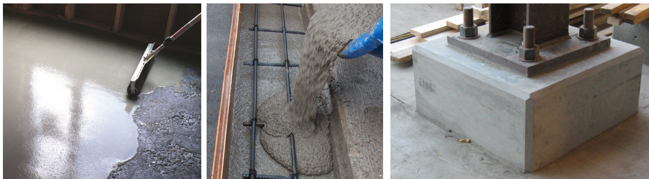
Figure 1: Cementitious components on site
